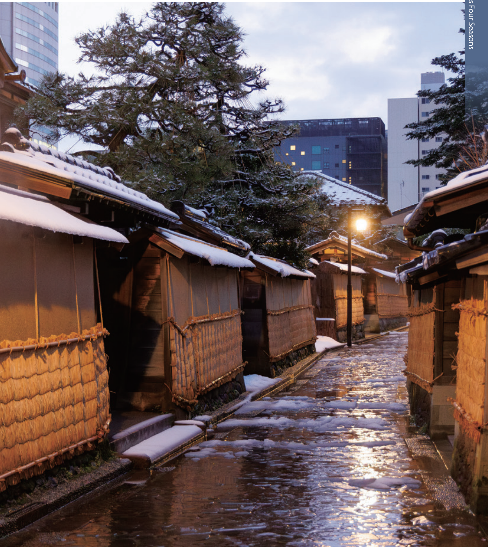
長町武家屋敷群の土塀の薦掛け Woven straw mats on the earthen walls in the Nagamachi samurai residence area
